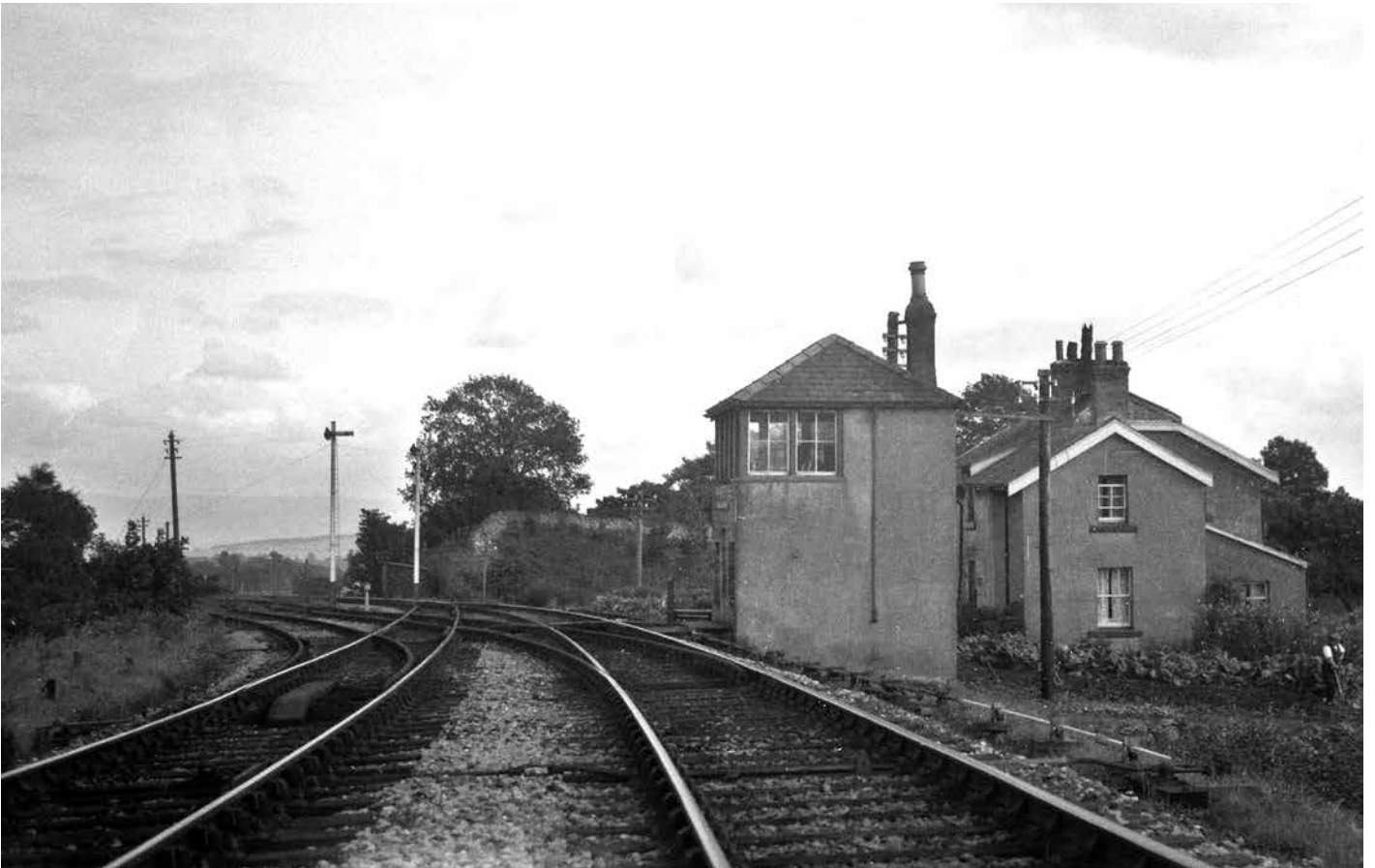
Redhills Junction looking east about 1935. The NER Redhills curve diverges from the CKPR off to the left. The line then descended to pass underneath the Keswick line and join the L & C at Eamont Bridge Junction. A closer inspection of the print reveals that the tops of the rails on the NER curve are dark with rust, indicating little or no use by this date.
